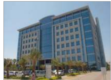
Delivery Centre III, Chennai (South India)
